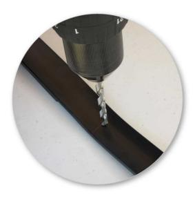
Use drill bit supplied, to drill holes in marked positions.
